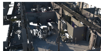
(h) Corridor view of the construction site from GT_4
