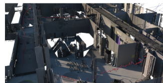
(f) Corridor view of the construction site from GT_3
