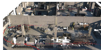
(g) Close-up view of the construction site from GT_4
