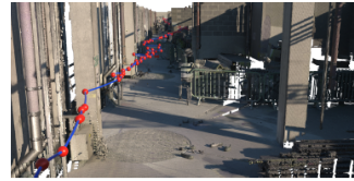
(b) Corridor view of the construction site from GT_1
