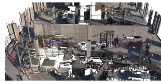
(a) Close-up view of the construction site from GT_1
